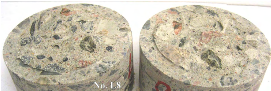
Figure A.45 Photograph showing the failure surface for test No. L8 after fatigue test.
